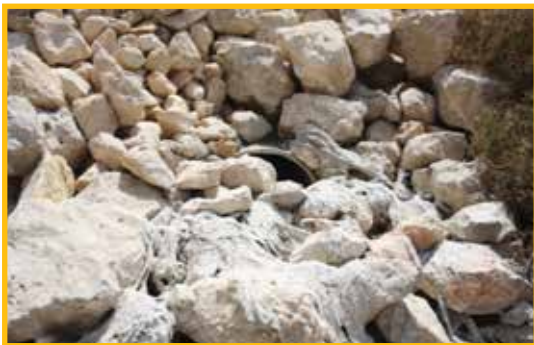
The wastewater pipe leading onto Wadi Foukin's lands complete with sewage remains.
